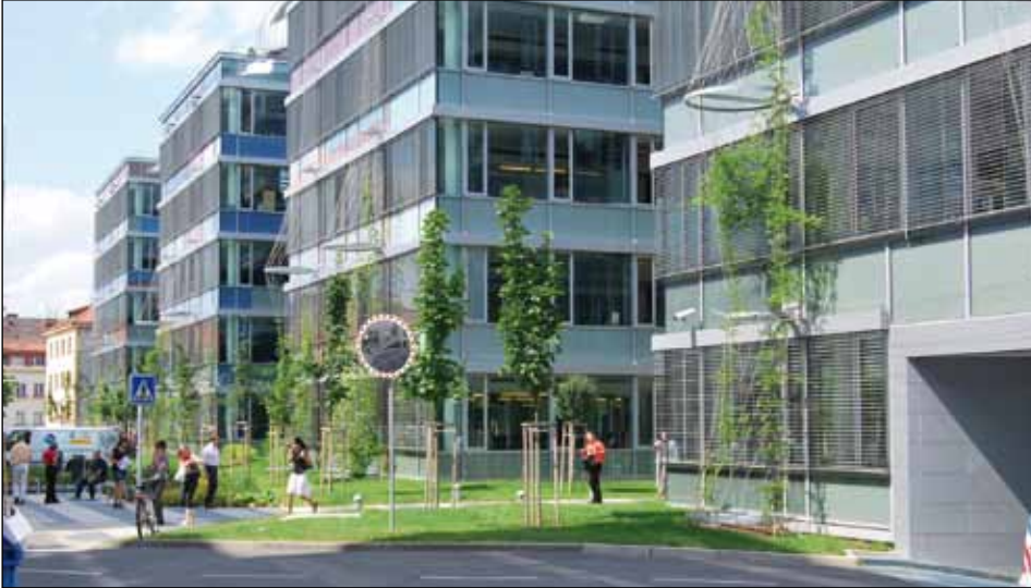
The sun protection systems controlled with KNX help to improve the energy balance considerably
