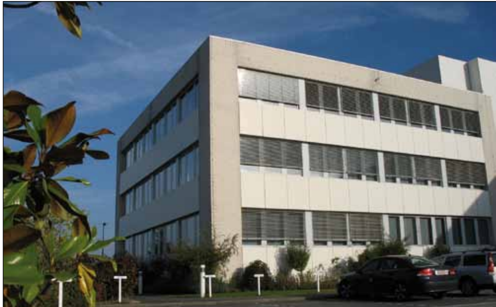
A sensor-controlled sun protection system reduces the cooling load
