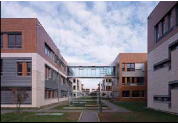
In the lighting installations between the building complexes, a clear energy saving potential can be opened up with KNX. Foto: Infineon/Heinemann
